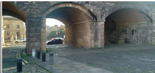
Designated assembly point
